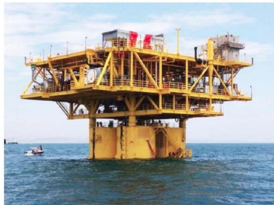
**Figure 2: Horton Wison Deepwater Buoyant Tower**
